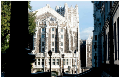
The City University of New York's City College campus at Broadway and 138th Street in New York.
